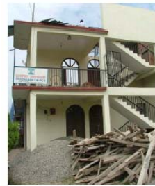
Building renovation—the way that it's done here!
