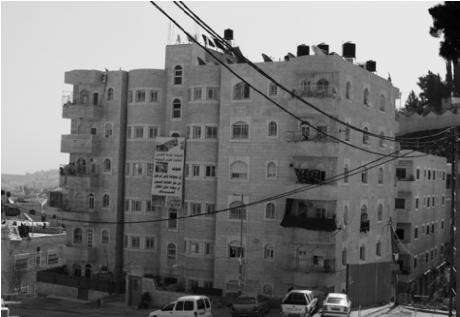
The two apartment buildings housing 34 families - 250 people - that received demolition orders on 5 March
